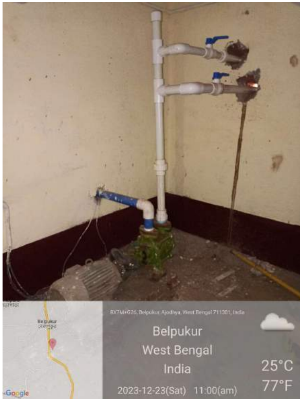
Pumping system from Rainwater reserve to OHR
