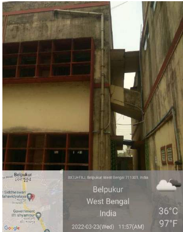
Rainwater outlet from rooftop to reserve
